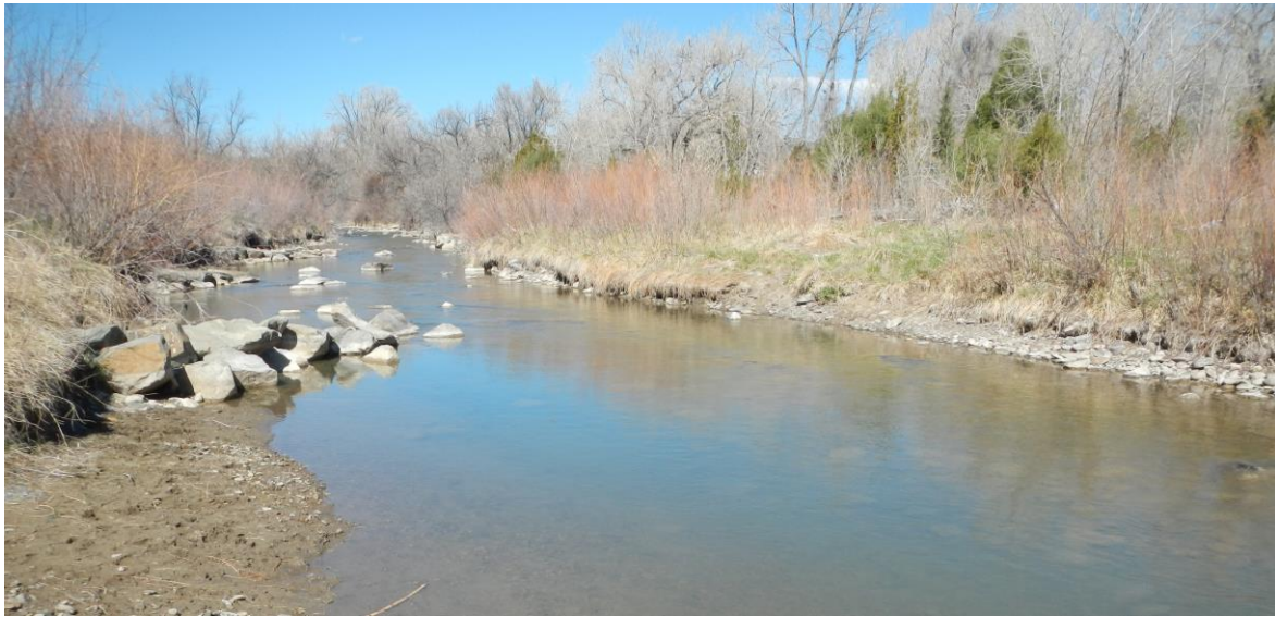
Boulder vanes and micro-vortex structures within the Purgatoire River study reach.
